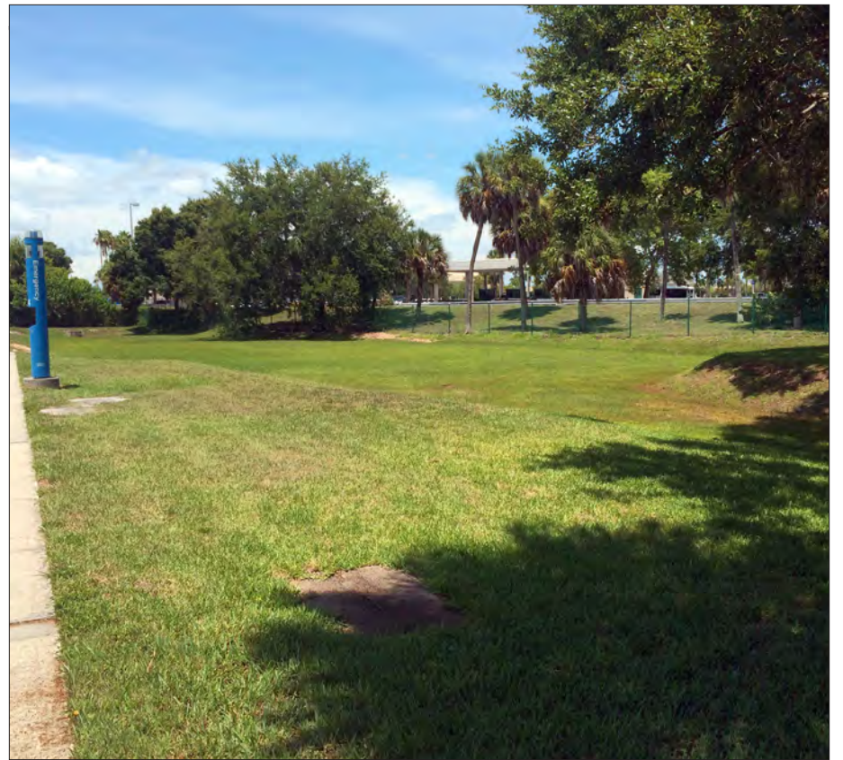
Dry Retention Pond near Airport
