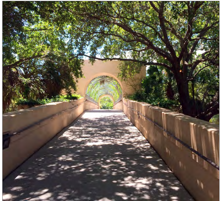
Pedestrian Bridge over US 41
